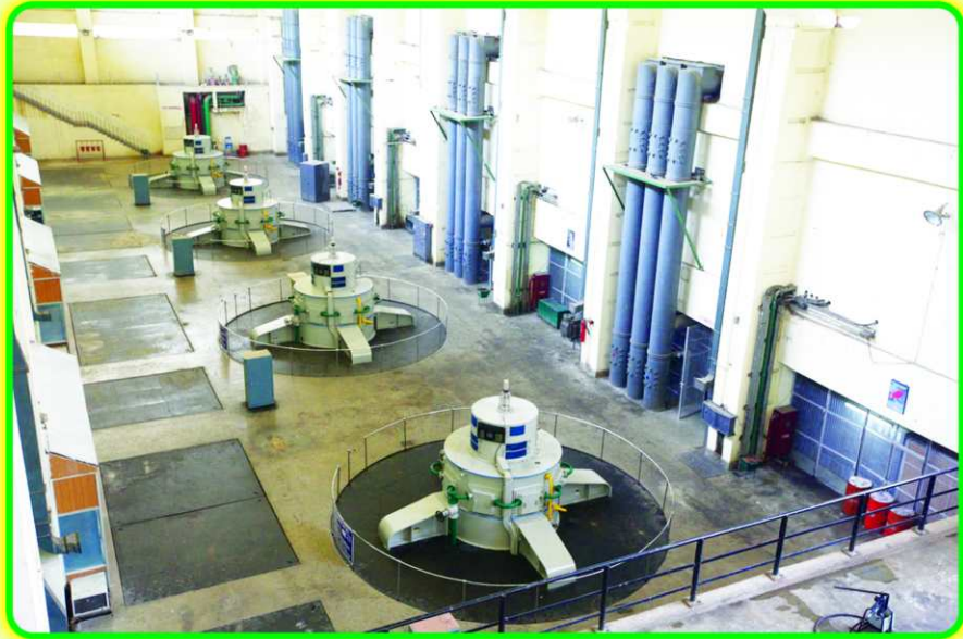
Generator Floor Upper Kolab Power House.
