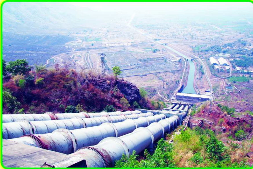
View from valve House Upper Indravati Power House.
