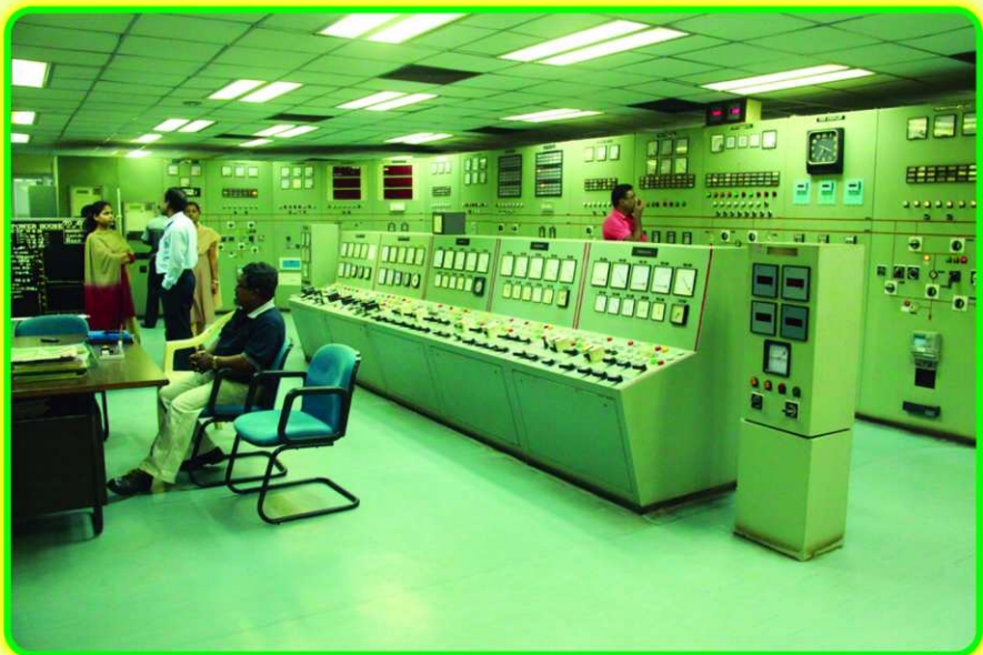
Control Room Rengali Power House.
