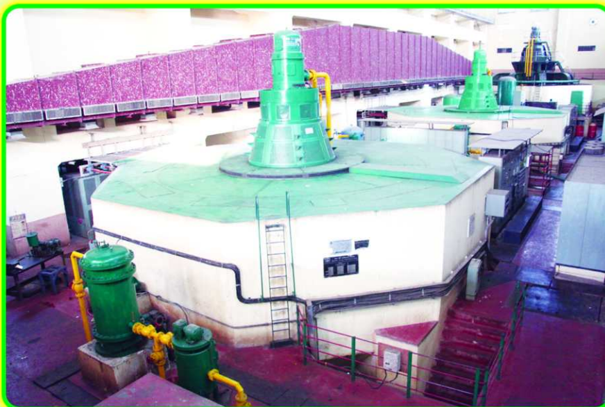
Chiplima Power House Generator Floor.
