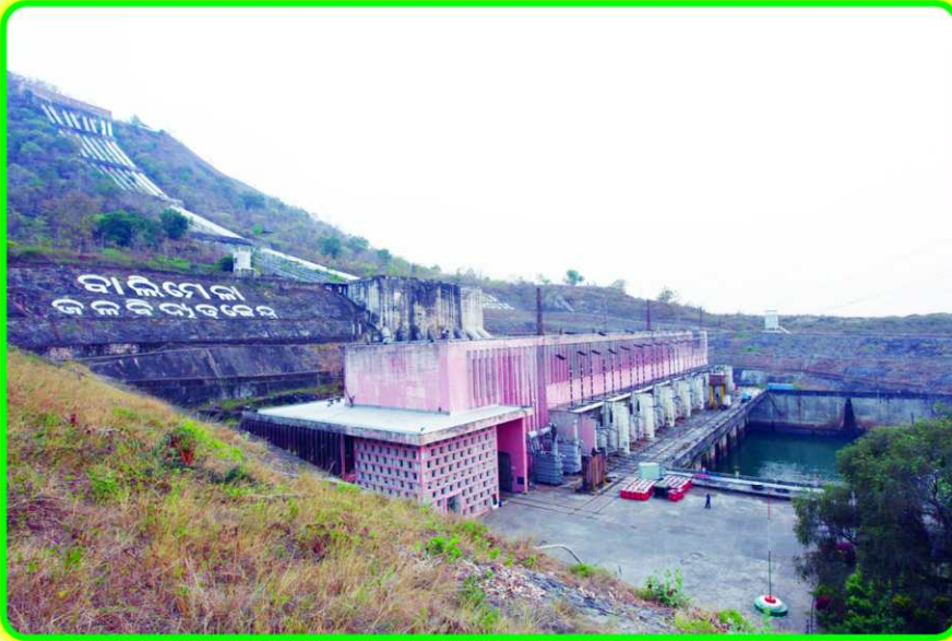
Balimela Power House.
