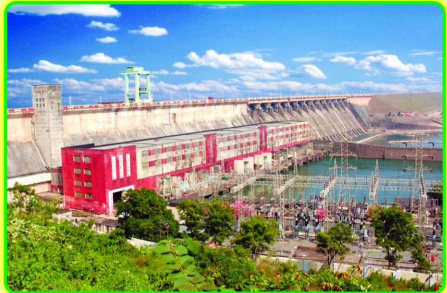
Hirakud Power House, 132 KV Switchyard.
